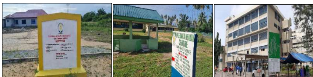
Figure 5.40 L-R: CHPS Compound (Sanzule), Health Centre (Ekebaku), Regional Hospital (Takoradi)
