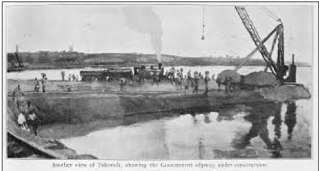
Figure 5.57 Construction of Takoradi harbour During 1920s
